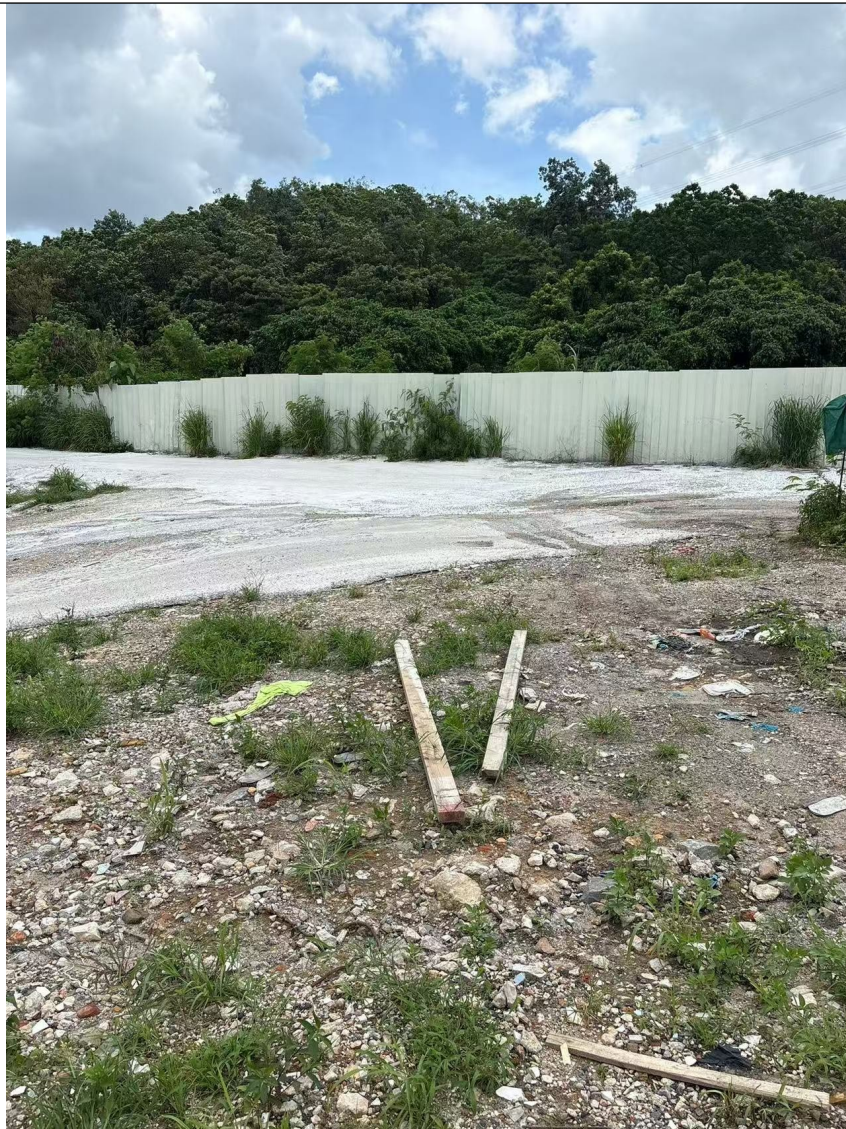
Photo 2: Existing site view and ground condition within the application site.
